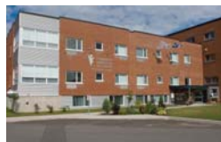
Mauricie Regional Centre and Lodge 456 residents 3,727 overnight stays
