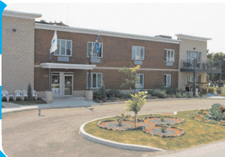
Outaouais Regional Centre and Lodge Michael J. McGivney Pavilion
