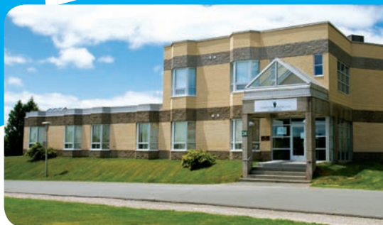
Estrie Regional Centre and Lodge
